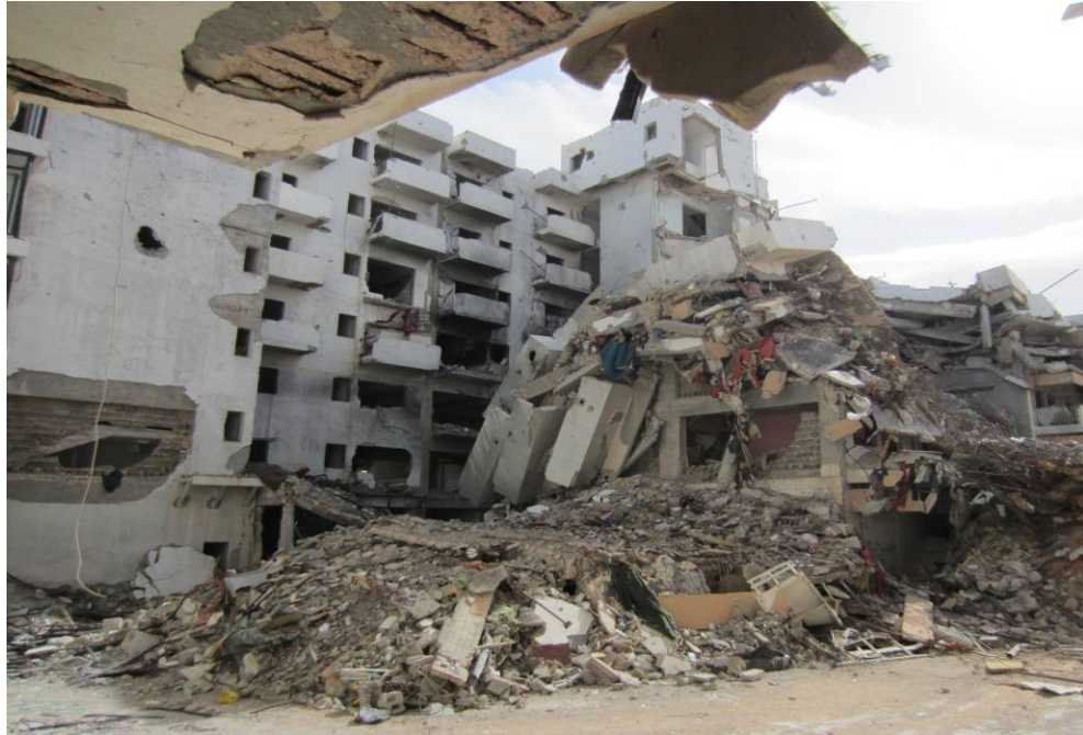
Apartment building struck on 16 September in Sirte © Amnesty International
